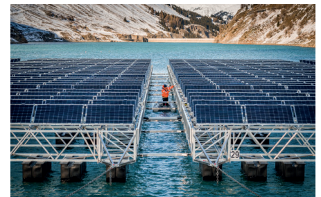
Installation of floating PV on a Swiss mountain lake ©Romande Energie
